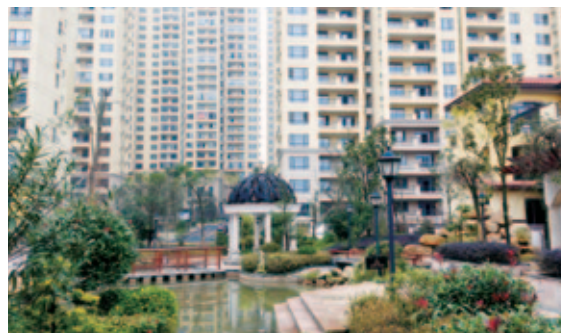
High-rise apartments of Tianyu-Huafu
